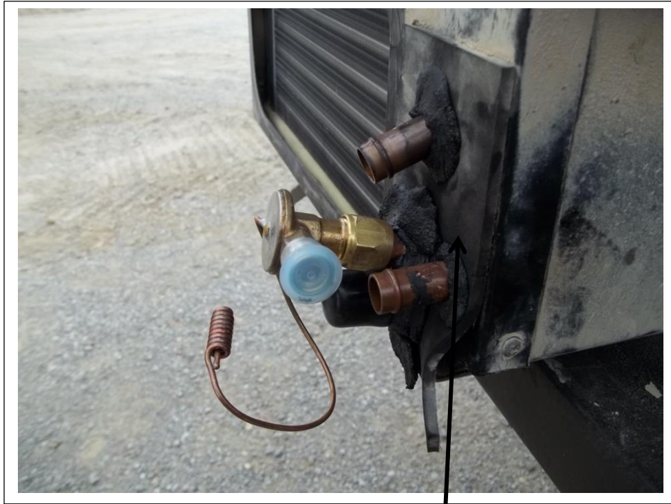
Seal all openings around the tubes with tar tape as shown.
